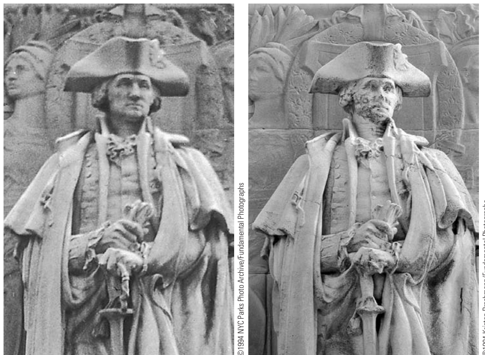
FIGURE 16.8 The calcium carbonate in marble and limestone is very slightly soluble in neutral water. Its solubility is much greater in acidic water. Objects carved of these materials dissolve relatively rapidly in areas where rain, snow, or fog is acidified from air pollution. Shown here is the damage to a marble statue of George Washington between 1935 (left) and 1994 (right).
