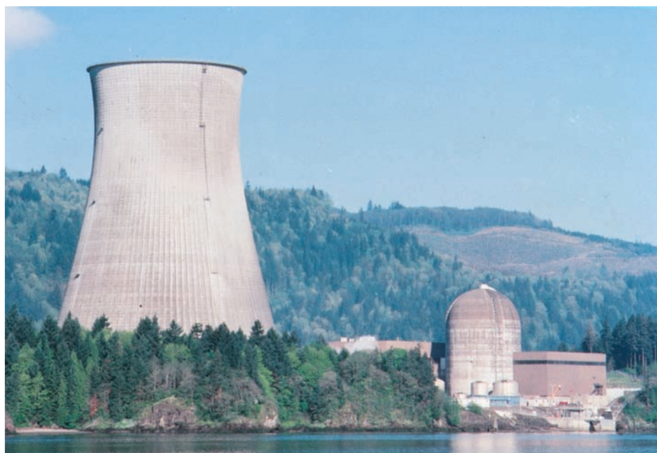
FIGURE 19.11 A nuclear power plant. The large structure on the left is a cooling tower; the containment building is the smaller building on the right with the domed top.
